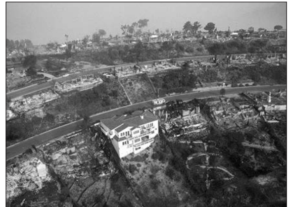
This house survived the 1993 fires in Laguna Beach, CA because of special design features and stucco cladding.
