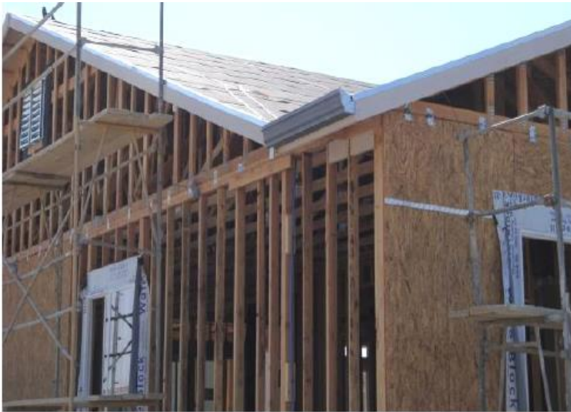
Figure 1: Sheathing only at shear locations
